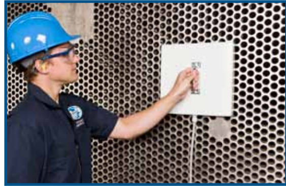
Tracer gas tube leak detection
