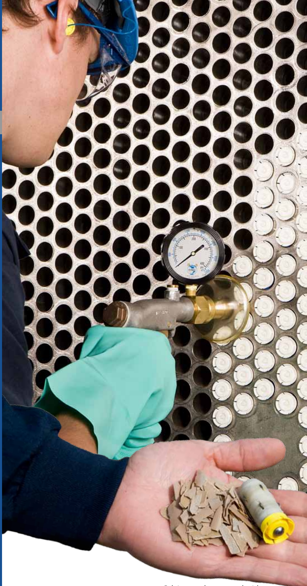
Calcium scale removed with Conco Calbuster
