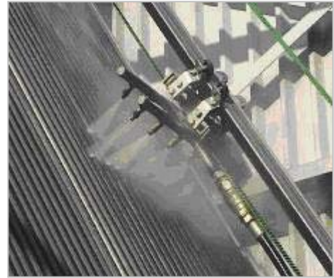
System nozzle head cleaning fins in a controlled, automated fashion
