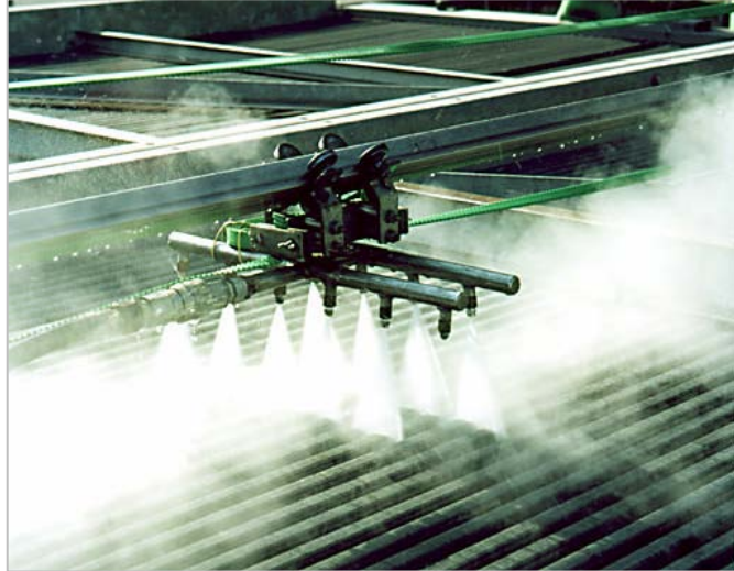
Conco FinTech™ Cleaning System cleans at 325 square feet per hour
